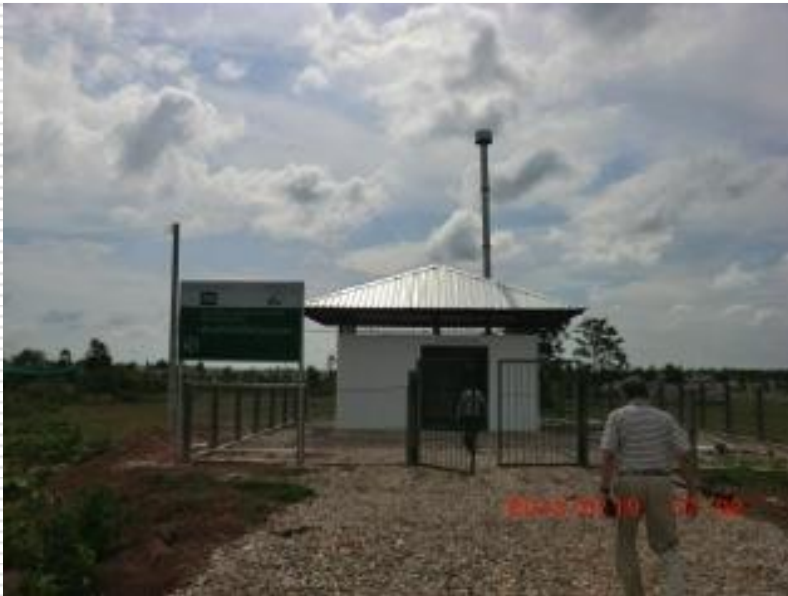
HCW Incinerator for Vientiane Capital
