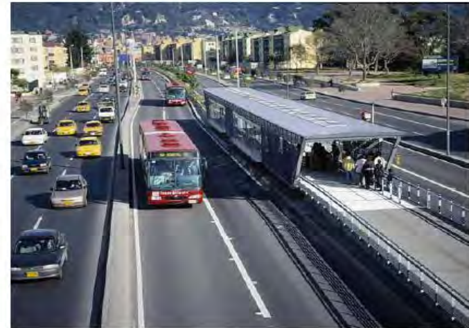
The TransMilenio BRT in Bogotá. Photo courtesy of Volvo Bus Corporation.
